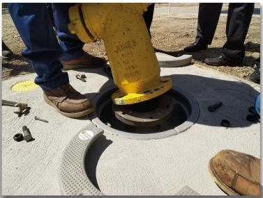
With no need to break concrete, the costs associated with fire hydrant repair are dramatically reduced.
